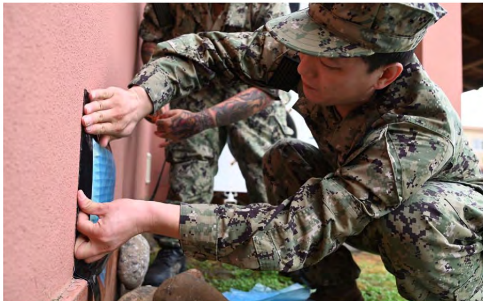
Petty Officer 2nd Class Zhijun Miao covers outside vents to prevent flooding of base housing units in preparation of a storm at Naval Air Station Sigonella, Italy, Oct. 28, 2021. Recent storms have flooded streets on base and impacted the power and drinking water supply in Sicily. (Kegan E. Kay/U.S. Navy)
