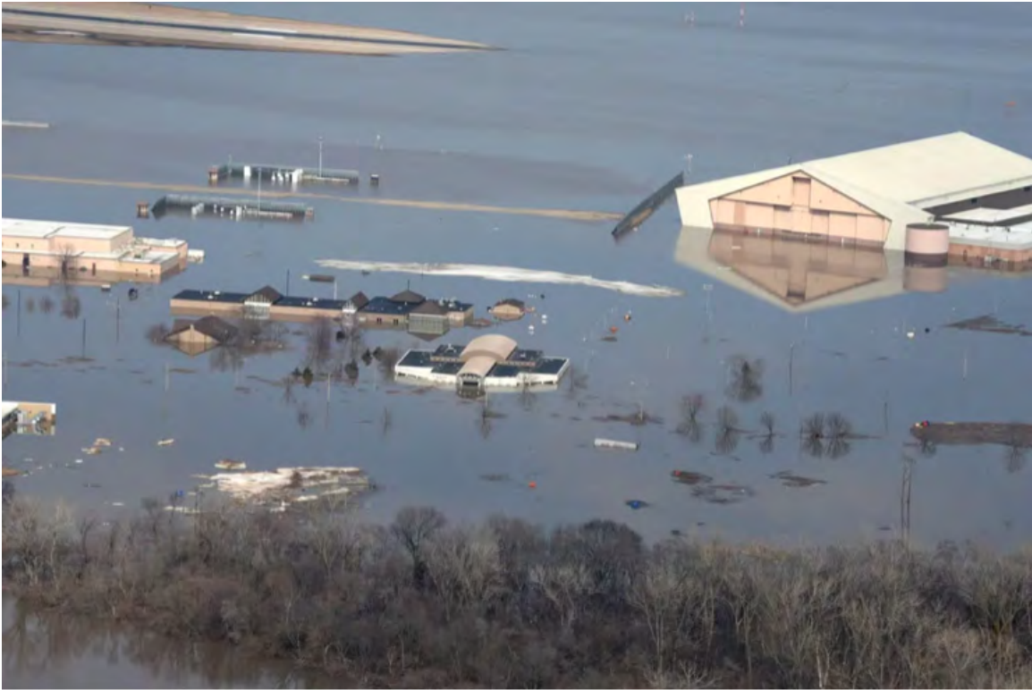
Figure 18. 2019 Missouri River Flooding at Offutt AFB. Severe flooding at Offutt AFB caused extensive damage to 137 buildings and inundated over half of the aircraft runway. Image accessed from: https://www.vox.com/2019/3/25/18280758/nebraska-flooding-air-force-offutt
