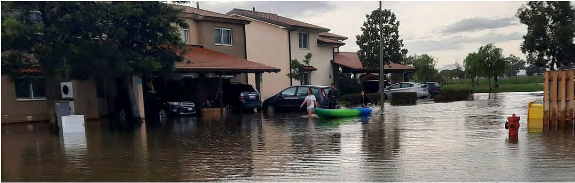
Figure 26. NAS Sigonella Base Housing Flooding after Rare Mediterranean Hurricane. Floodwaters inundated the Marinai housing complex because of power outages, pump failures, and floodwaters over-topping the levees. Image accessed from: https://issuu.com/nas_sigonella/docs/05nov2021/s/13998869
