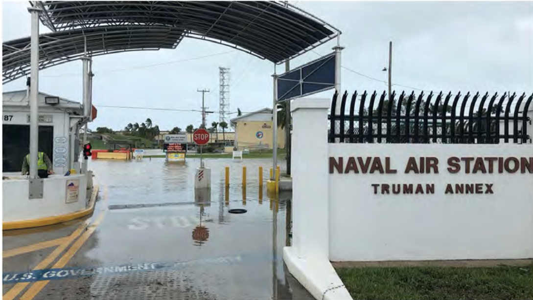
Naval Air Station Key West's Truman Annex experienced heavy flooding after an estimated 6 inches to a foot of floodwaters soaked through military housing and other base infrastructure. US Navy photo by Mass Communication Specialist 2nd Class Nicholas V. Huynh.
