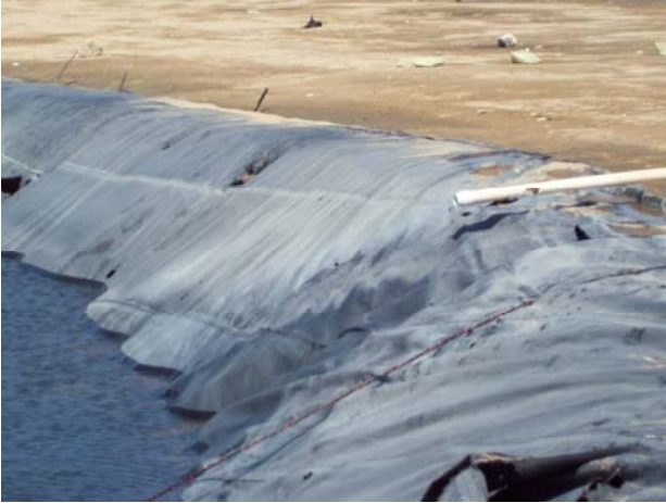
Figure 16. Ground water from a PVC pipe fills the test pond
