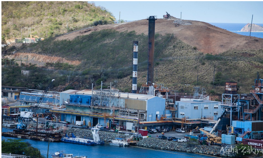
Figure 2. Harley Power Plant. Photo: VI Consortium.
