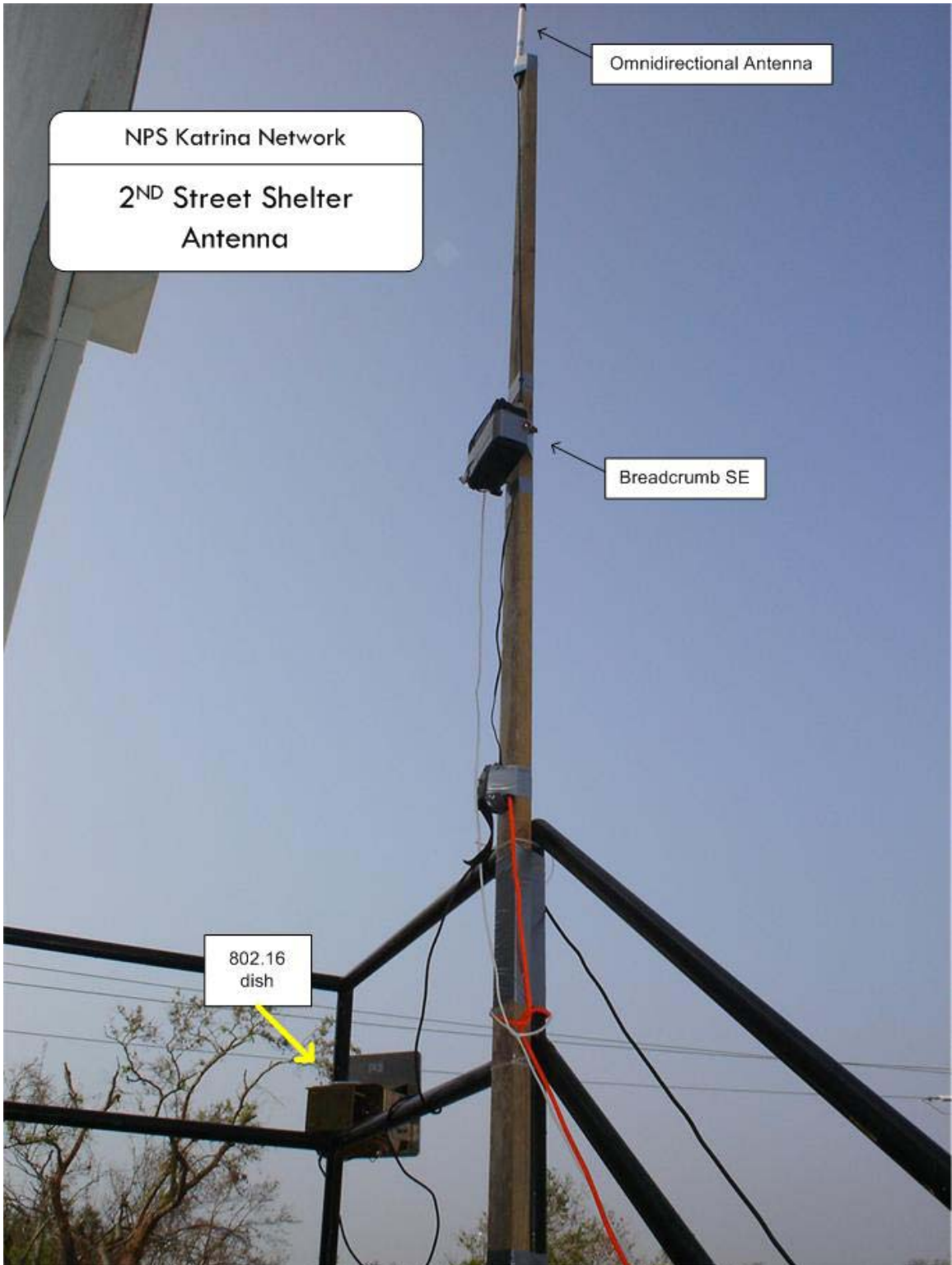
Figure 16. 2 nd Street Elementary School Shelter Antennas (as of 19 September 2005)
