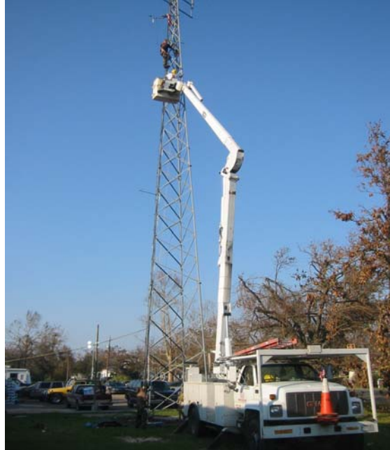
Figure 6. NPS Student on Power Company Bucket Truck Installing 802.16 Gear in Bay St. Louis on Surviving Antenna Tower
